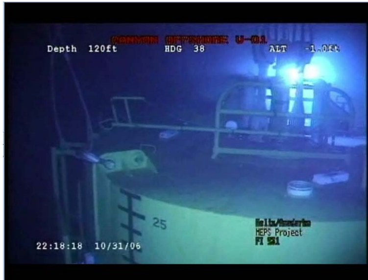
Fig. 11 ABC SSR Installation after Two Years of Service in Gulf of Mexico
